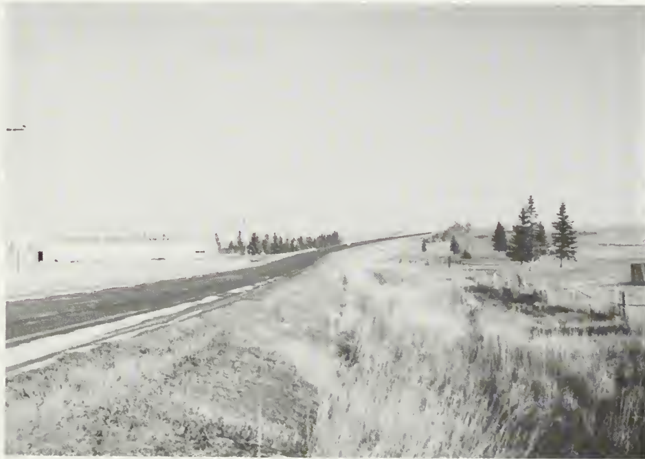
Figure 1 - North view near milepost 0.4
